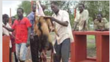
Slaughter facilities are constructed to improve meat quality and marketing - Malakal upper Nile
