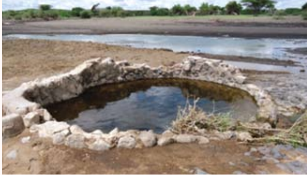
Destroyed (unprotected) shallow well along the river bank at El Waano before drainage and de-silting.
